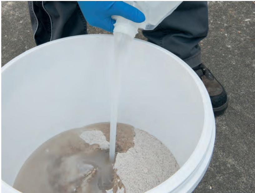
Giet vermengde Poxycon hars in de emmer op Poxy Quartz
